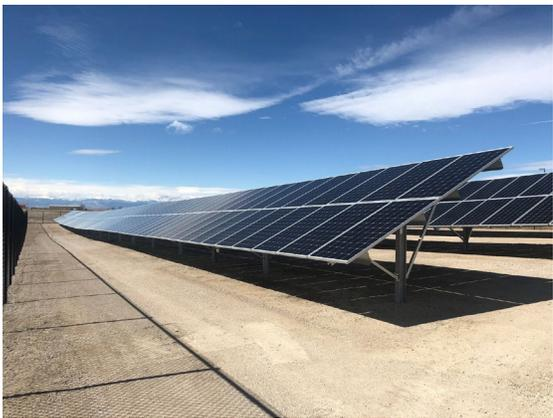
A newly installed photovoltaic solar system on Colorado’s Fort Lupton Readiness Center absorbs and converts solar energy, July 2020. The Colorado Department of Public Health and Environment’s Supplemental Environmental Program funded the 150kW Photovoltaic Solar array at the Fort Lupton Readiness Center in Colorado. Electricity generated by the solar panels will offset 100% of the facility needs which makes the Readiness Center Net-Zero electric.
